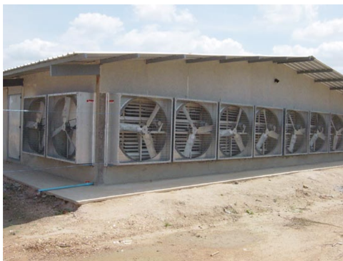
Figure 19: An Example of Power Ventilation
